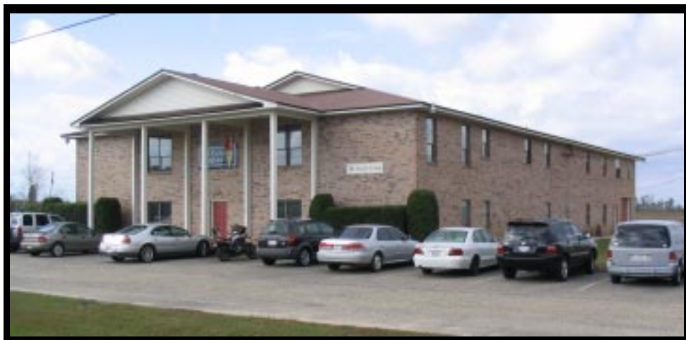
The landmark We Care headquarters building, erected in 1984, to be vacated by April 1, 2006
